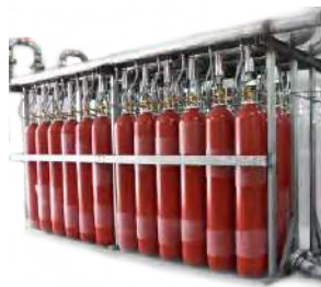
CO2 Extinguishing System
